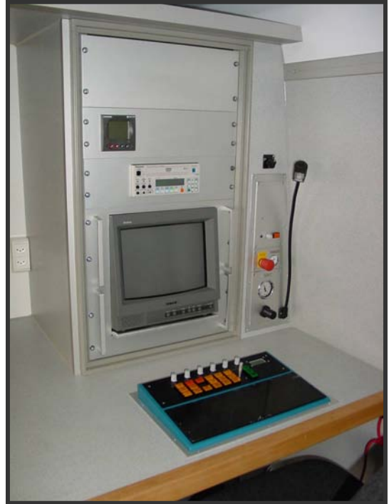
Cockpit: Controls, Monitor, On-Screen-Data, DVD Recorder
